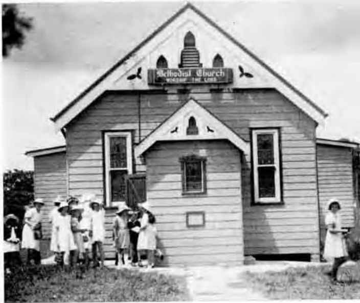
The original weatherboard Church as it appeared in 1941 after the additions had been completed.
