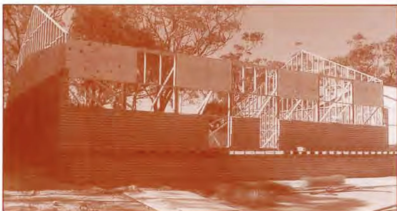
The new library during construction in 1994.
