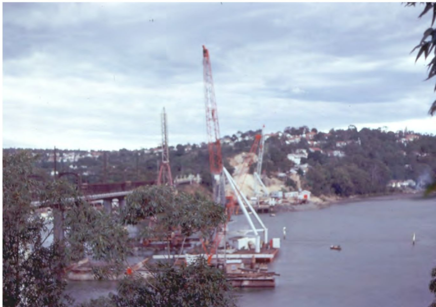
Approx. Early 1970 Work underway on the new Dual rail bridge
