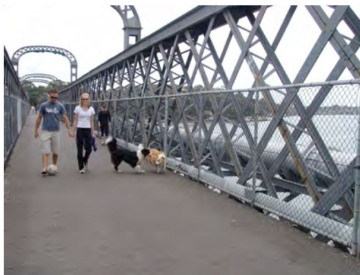
The cycleway / walkway is popular. Particularly at weekends.
