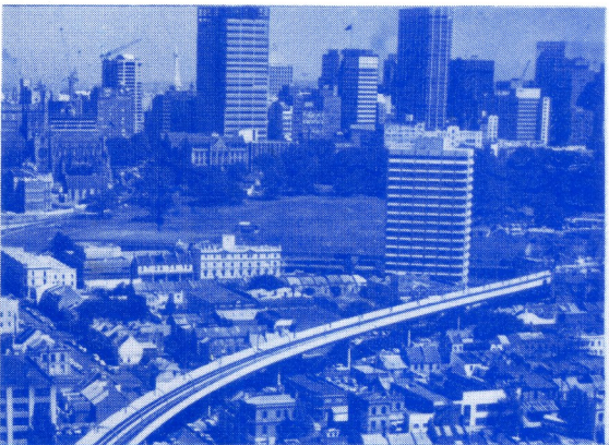
The Woolloomooloo Viaduct — Eastern Suburbs Railway.
