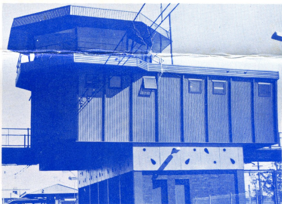
Modern signal control room overlooking Campbelltown rail yards.
