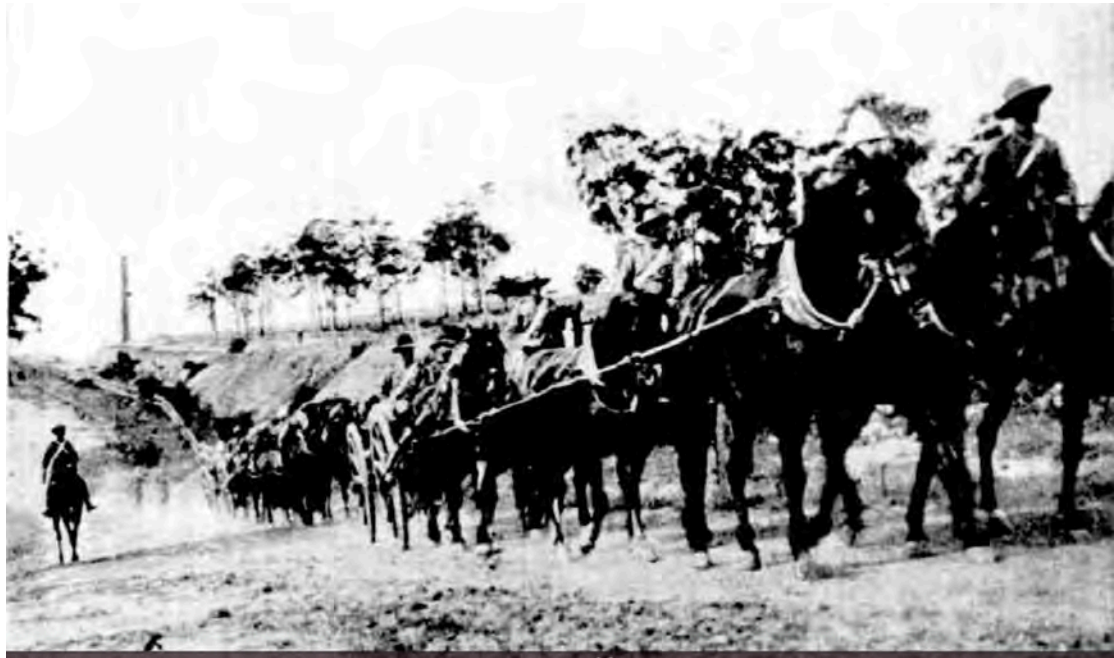
Photo of Oatley Parade with Embankment clearly shown and Mortdale brickpits chimney in the background. 1901.
