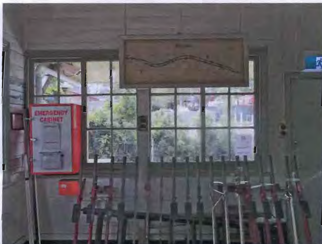
The preserved Signal Box at Oatley in 2017. The diagram shows the layout after the Engine Siding and Carriage Siding were removed. John Oakes.
