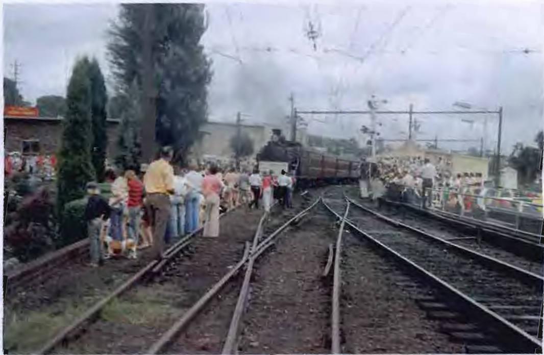
Oatley looking south on the occasion of the 50 th Anniversary of electric trains on 29 February 1976. RRC010183.
