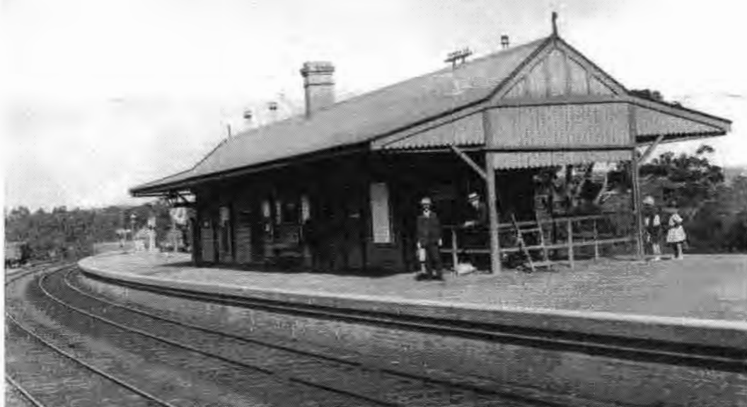
Oatley. The 1905 Oatley Station. The line on the left is the Engine Siding and the wagon in the background is on the Goods Siding. John Newland Postcard Collection RRC 510285
