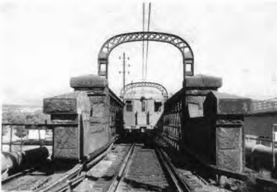
Looking south towards the Old Como Bridge in 1972. Note the gauntlet track.
