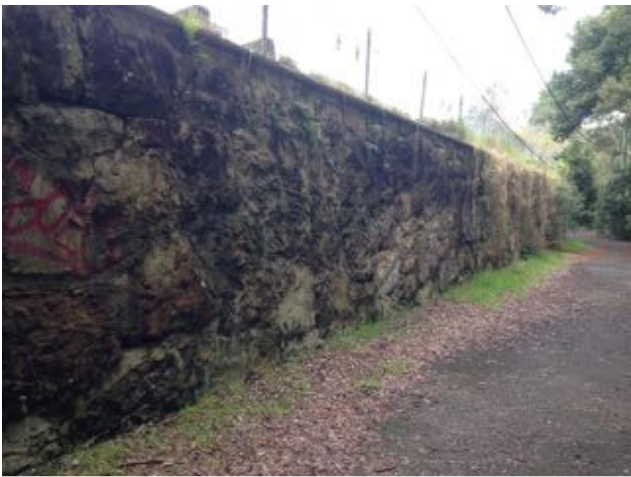
Lower no 2 green retaining wall.
